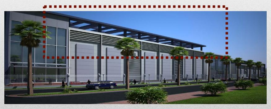
We try to find some design parameters related to the spacing, size, angle as even material of the sun shades. The objective will be a function with time and complexity required to solve the problem. One can even use rcontrib to calculate annual contribution of the sky/sun on the roof surface given a certain configuration
